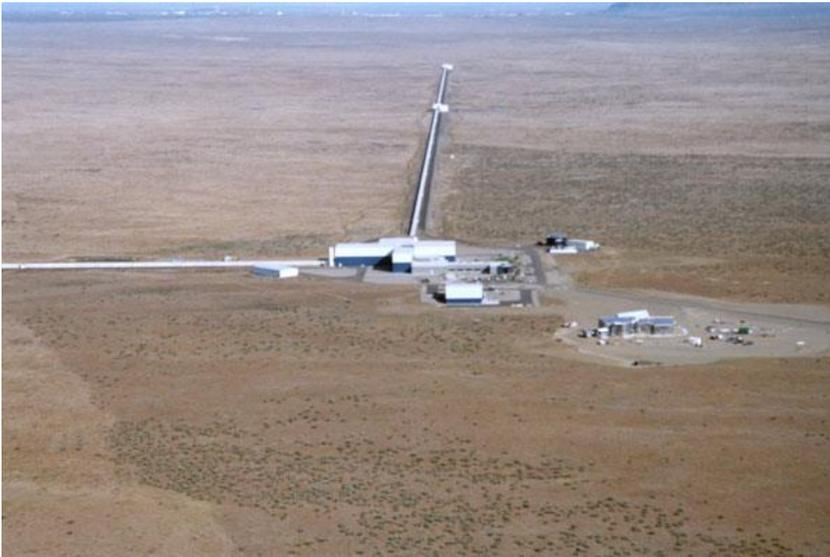
LIGO consists of two L-shaped interferometers, one in Hanford, Washington (shown here), and one in Livingston, Louisiana. Each arm of each L is 2½ miles (4 km) long. Lasers look for changes in each arm's length as small as a millionth the diameter of a proton. Passing gravitational waves might distort space-time by that much. *LIGO Laboratory*
