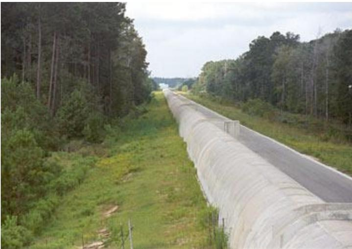
The tunnel for one of the LIGO arms in Livingston, Louisiana. Having two units nearly 2,000 miles apart provides essential error checking and would help triangulate to find the incoming direction of any gravitational waves. A third detector in Italy, named [VIRGO](#), is scheduled to join the network. *LIGO Laboratory*.
